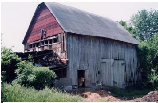
Duderstadt Barn, Warren Township, Somerset County - National Register nomination.
